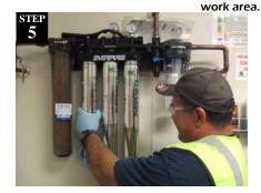
Remove three main filters by hand by turning a ½ turn. Properly dispose of used filters. Install three new filters by hand with approximately ½ turn until positive stop. Inspect O-Ring seals on both prefilter and filter. Replace as needed. Write the date on the filter, may use tape on cover.
