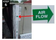
Insert new filter with proper orientation for air flow. Air flows in the direction of the radiator. Lock panel back in place with using all screws/levers. Clean work area.
