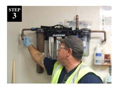
Close main water valve upstream of filters. Open bleed valve to relieve water pressure and drain water into sink.
