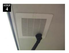
Vacuum return air grill of any dust and debris. Wash with soap and water if debris cannot be vacuumed off. Clean work area and return sign to store sign kit.
