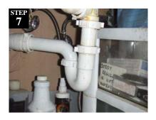
Hand tighten plastic nuts to secure trap back in place, run water to test for leaks, and remove inoperable sign and floor signs. Clean work area.
