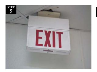
Example of faulty EXIT sign is dark, but lights up when "Test Button" is pressed.
