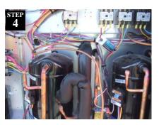
Visually inspect wiring for blown or loose fuses. Close panel and turn power back on to unit.
