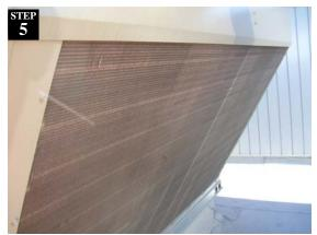
Spray with water nozzle perpendicular to fins. Spraying at an angle may bend the fins. Do not use a coil cleaner unless dirt is "caked on." Turn power on.
