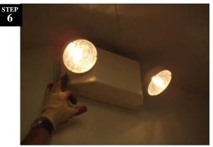
Example of Emergency Lights only kit lit up with the Test Button. Replace signs as needed.
