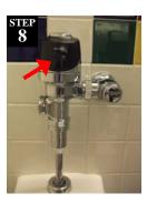
Reinstall the electronic flush unit and secure it with the locking ring. Clean automatic flush sensor window with damp rag. Clean work area. Return sign to store sign kit.
