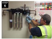
Unscrew scale reducing cover by hand. Remove and properly dispose of used scale reducer element. Rinse cover with clean water and wipe with clean towel. Install new scale reducer element inside cover and screw on by hand until tight. To reduce algae growth, please furnish and install: EV 6500-22 Filter Bowl Sleeve 10" Blue or EV 6500-23 Filter Bowl Sleeve 20" Blue.
