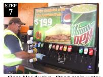
Close bleed valve. Open main water valve. Check complete filter assembly for leaks. If no leaks, open bleed valve and flush entire filter system for at least 5 minutes. Close bleed valve after flushing. Plug in fountain carbonator pump. Check all foodservice equipment for operation and remove signs. Clean up work area.
