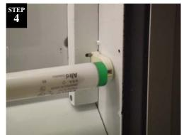
Twist lamp to align prongs with slot and remove. Dispose of lamp in broken lamp box supplied by Sylvania. Do not leave lamp on ladder or near customer's path to install new lamp.
