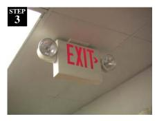
Check exit sign to ensure "EXIT" letters are illuminated. (Good EXIT sign with emergency lights.)
