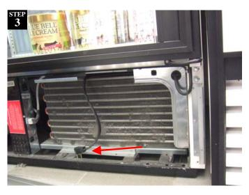
Unplug electrical cord (see red arrow). Vacuum all dust and debris being careful not to bend the fins on the coils. Plug unit in. Remove barricades and clean work area. Return "Cleaning in Progress" sign to sign kit.
