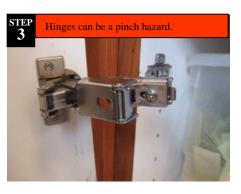
If door will not shut appropriately then use the screws to adjust the hinge.
