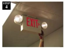
Check emergency lights with test button. (Good EXIT sign with emergency lights lit up with Test Button.)
